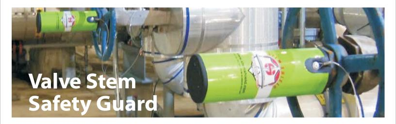
Stem Shields provide simple, cost-effective safeguards against the all-too-preventable injuries sustained when workers bump, graze, or ram into stems that project from industrial valves.
