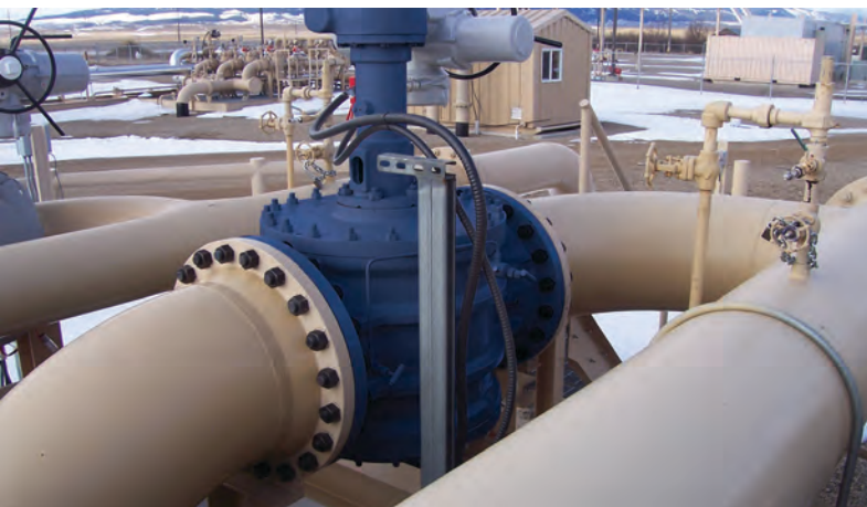
OmniSeal® DBB expanding plug valves in service
