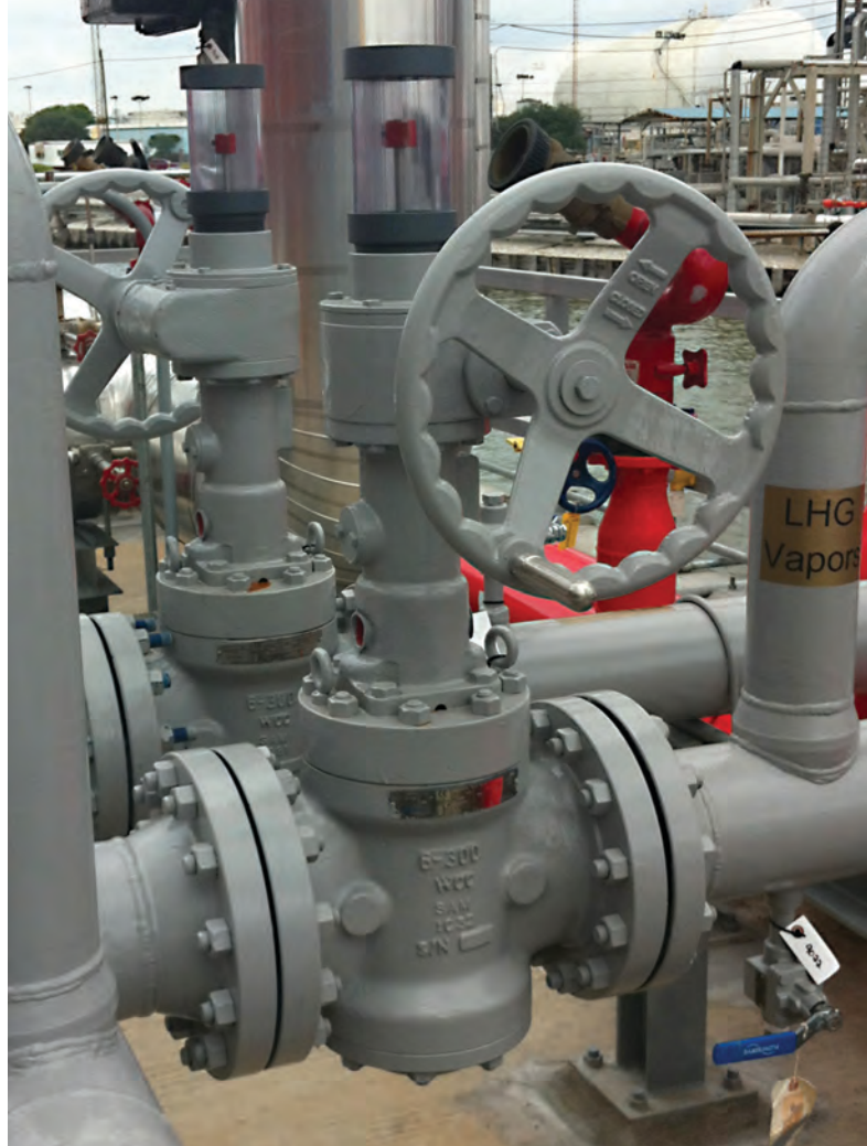
OmniSeal® DBB expanding plug valves during installation
