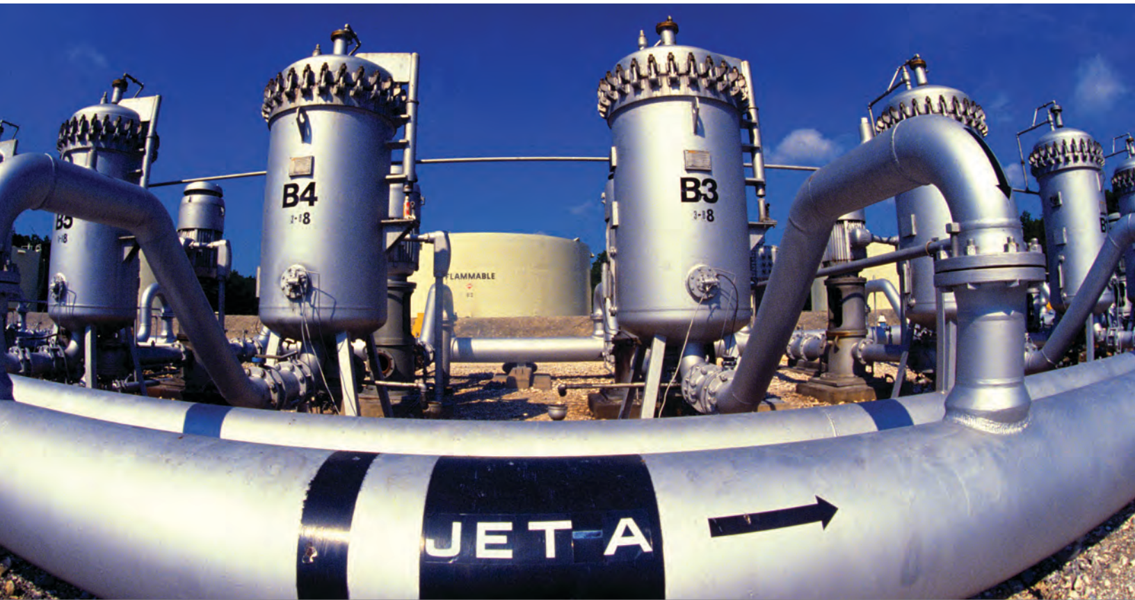
OmniSeal® DBB expanding plug valves in service
